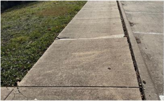
Lift parking lot sidewalk to eliminate cross-slope tilt
