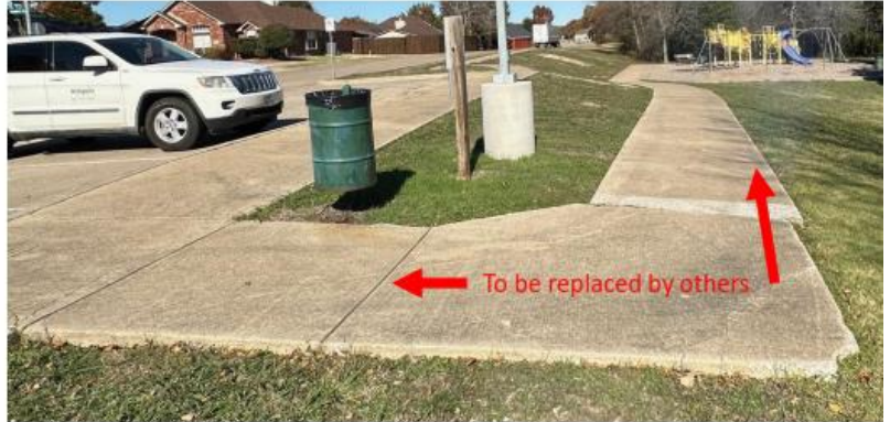
Lift sidewalk to eliminate cross-slope tilt
